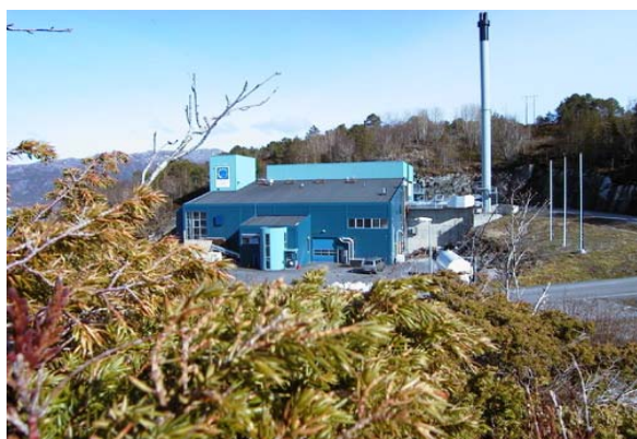
Photo: A Gasification plant, Norway
