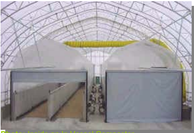
Photo: Inside an In Vessel Composter
