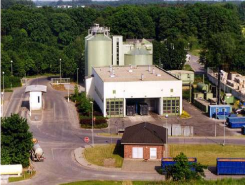
Photo: Anaerobic Digester
